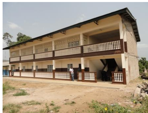
The Henri Williams Memorial Building which houses the three laboratories
